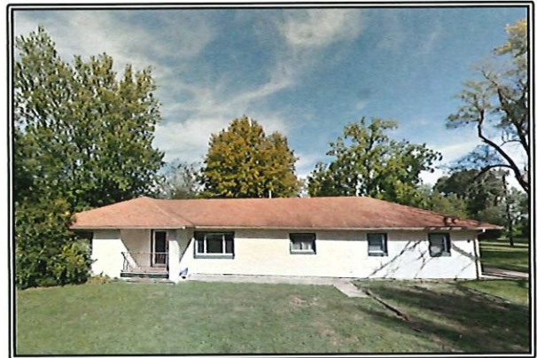
201 North Park Street
