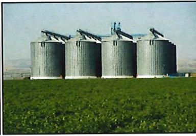
Grain Storage Facility
