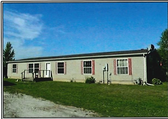
713 South Lafayette Street
